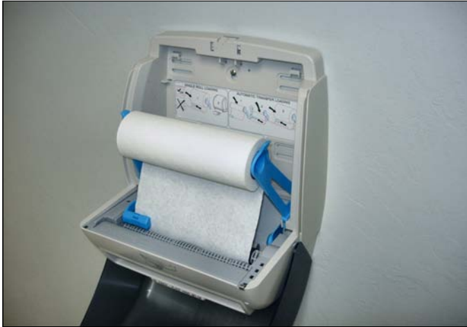
When the roll of paper is at 3" Dia. Or smaller, it is time to replace it with a new roll.
