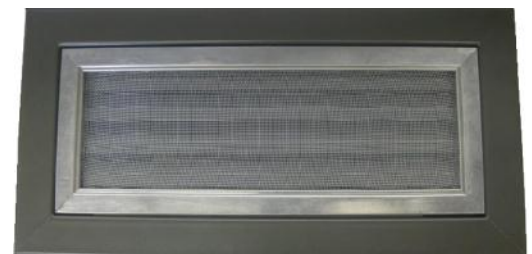
18 x 14 mesh insect screen installed
